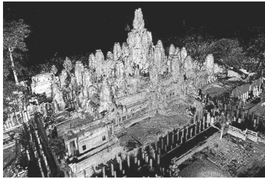
Figure 19.3. measurement result of entire Bayon temple
